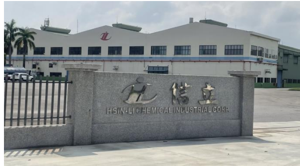
Syuejia District Factory Four(Occupying 13,394 tsubo)
